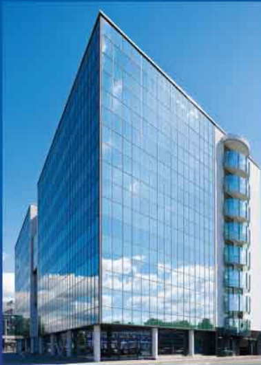
Primium Office Building, location: St. Petersburg, completion: 2007...2008
